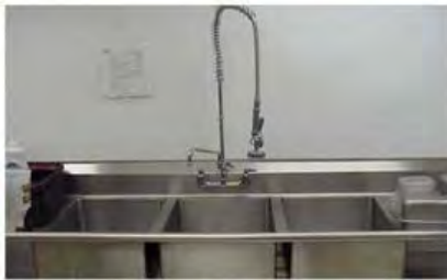
Figure 7: Three-sink dishwashing system.
