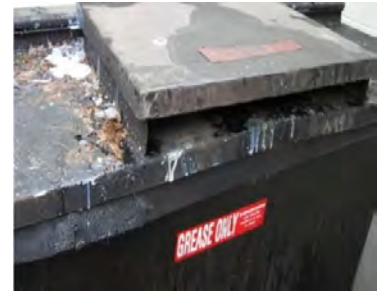
Figure 31: Spills on and around grease recycle bin.
