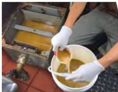
Figure 19: Removing grease from the grease trap.
