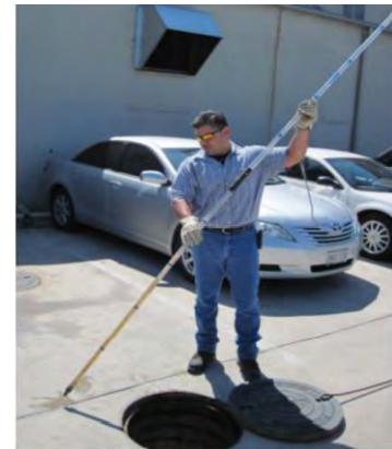
Figure 25: Inspecting the interceptor.
