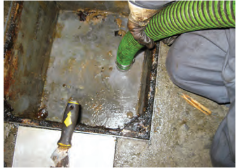
Oversee contractors for complete, correct service.
