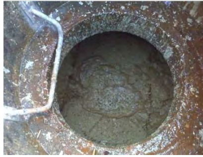
Figure 23: View into a manhole on the interceptor inlet.
