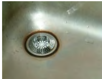
Figure 8: Sink drain screen.
