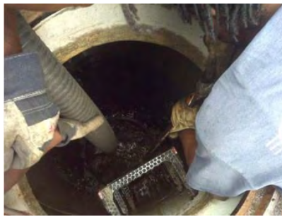
Figure 27: Use of high pressure water and suction hose.
