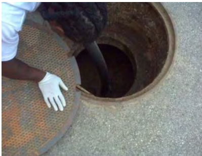
Figure 26: Vacuuming out the contents of the interceptor.
