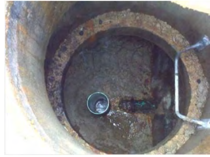
Figure 24: View into a manhole on the interceptor outlet.
