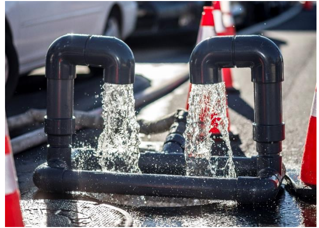
Figure 2. Baffle draining system.
