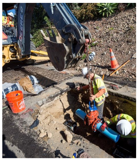
Figure 3. Our team replacing a valve.
