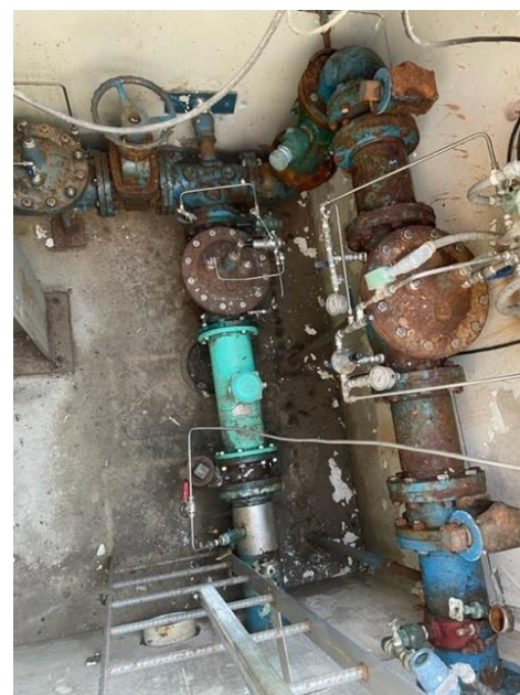
Figure 4. EOCWD historical image of Hewes Vault.
