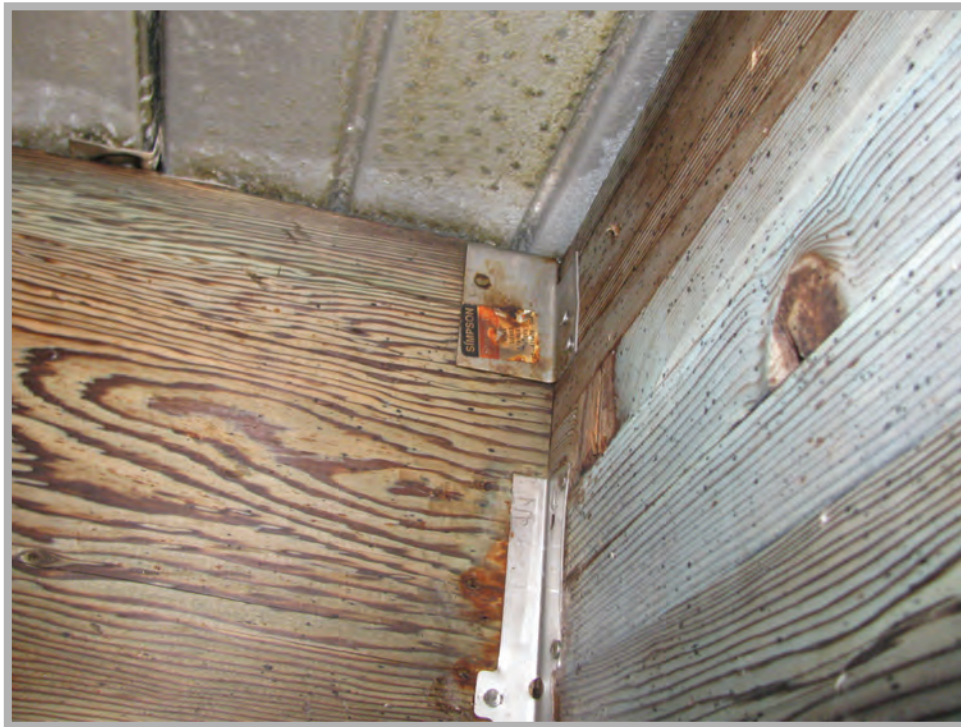
Photo B.11 Peters Canyon Reservoir Purlin to Glulam Connection
