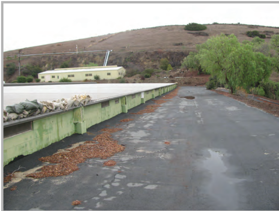
Photo B.16 Peters Canyon Reservoir South Wall Looking North-East
