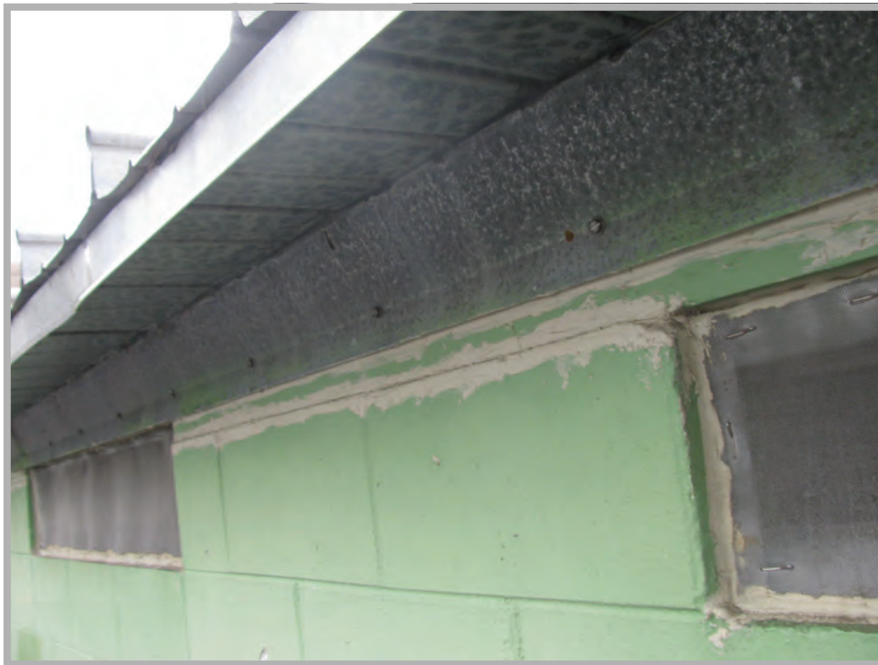
Photo B.6 Peters Canyon Reservoir - Typical Roofing and Flashing
