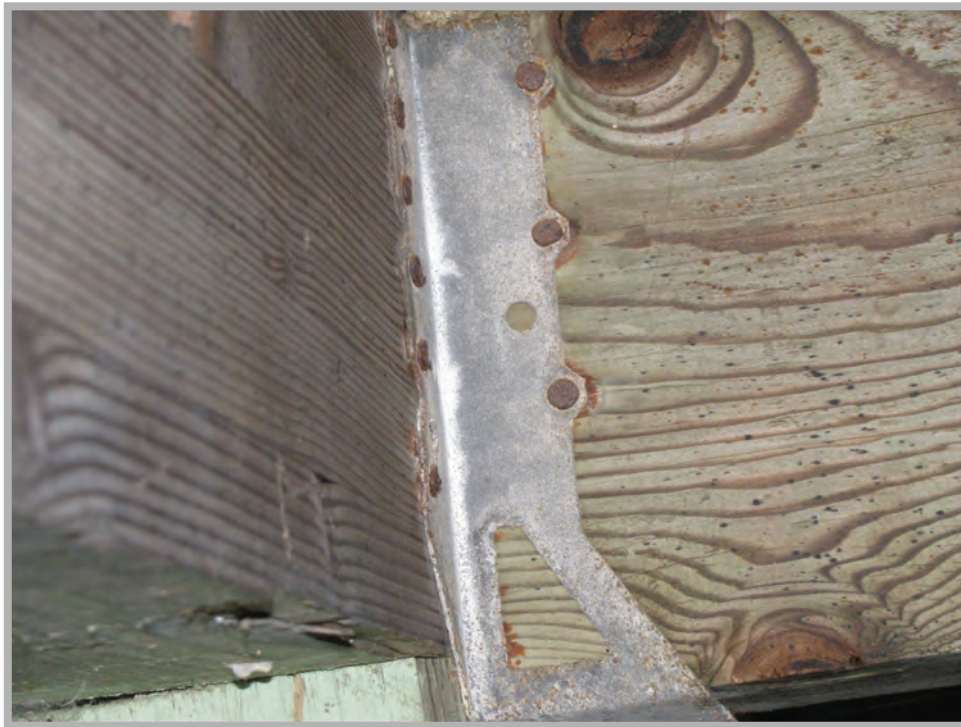
Photo B.15 Peters Canyon Reservoir Typical Hanger Connection at Purlin
