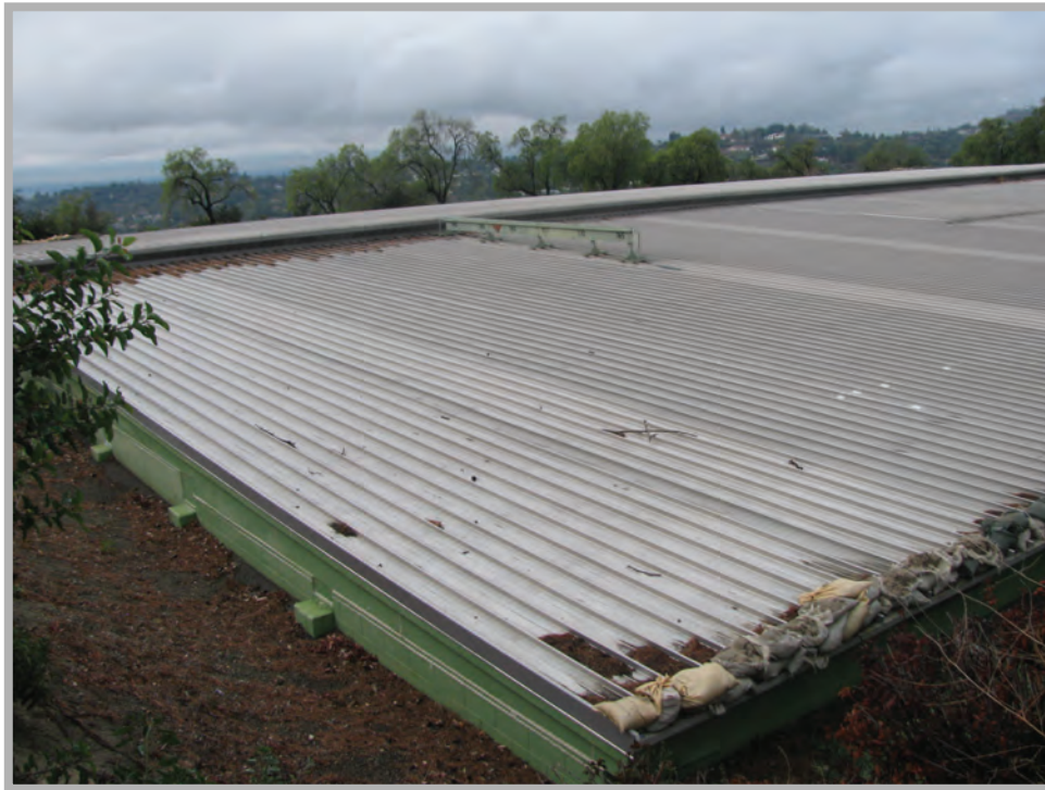
Photo B.1 Peters Canyon Reservoir Roof Looking South West
