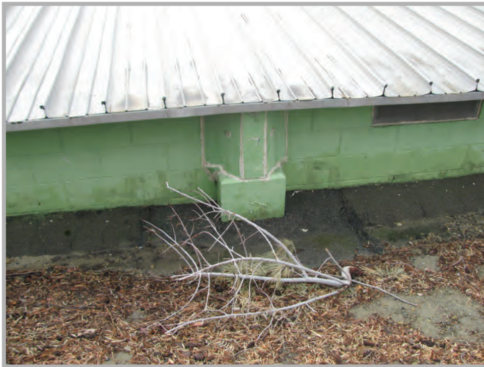
Photo B.4 Peters Canyon Reservoir Typical Pilaster
