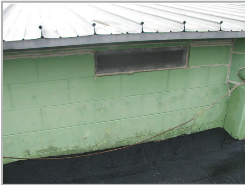
Photo B.5 Peters Canyon Reservoir CMU wall Vent and Zip-Rib Roof
