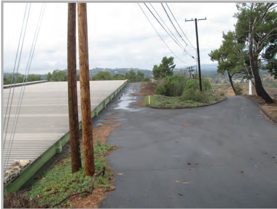
Photo B.2 Peters Canyon Reservoir Roof and North Wall
