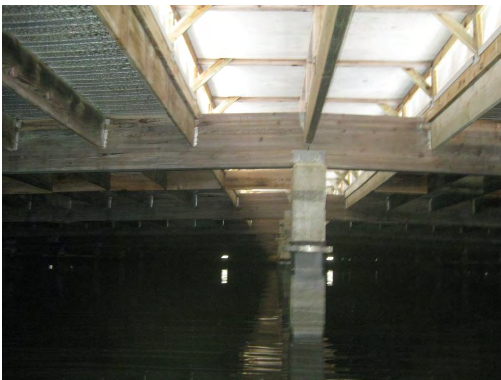
ROOF FRAMING AT CENTERLINE OF RESERVOIR
