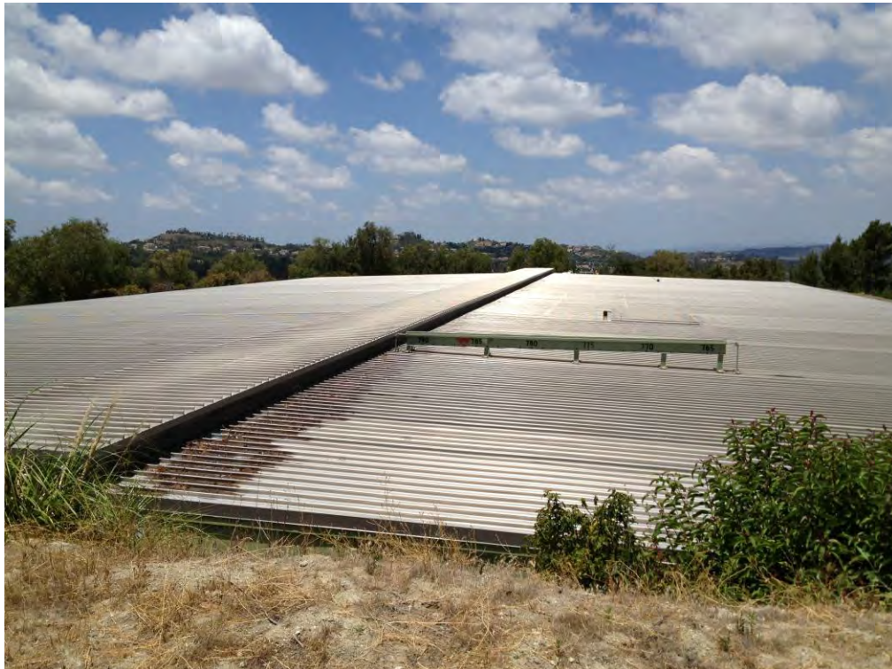
OVERALL ROOF LOOKING WEST
