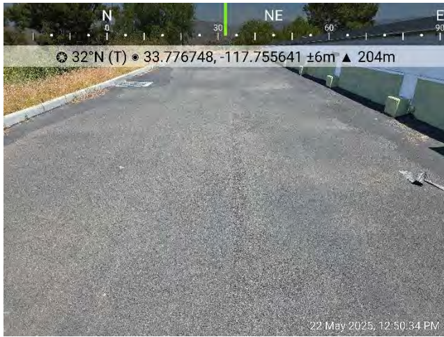
view: Asphalt surface along the west end of the site
