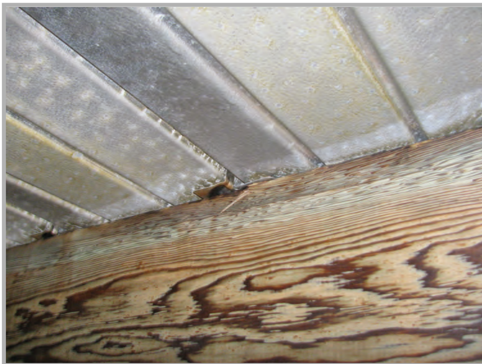
Photo B.14 Peters Canyon Reservoir Zip-Rib Interior Clip Connection
