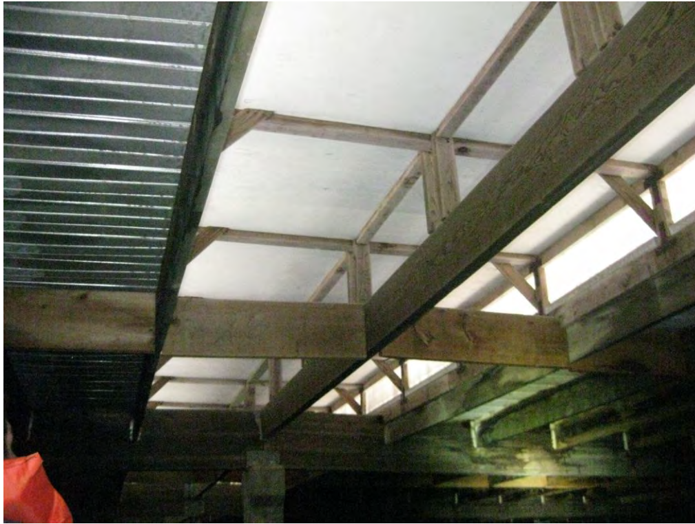
ROOF VENT FRAMING
