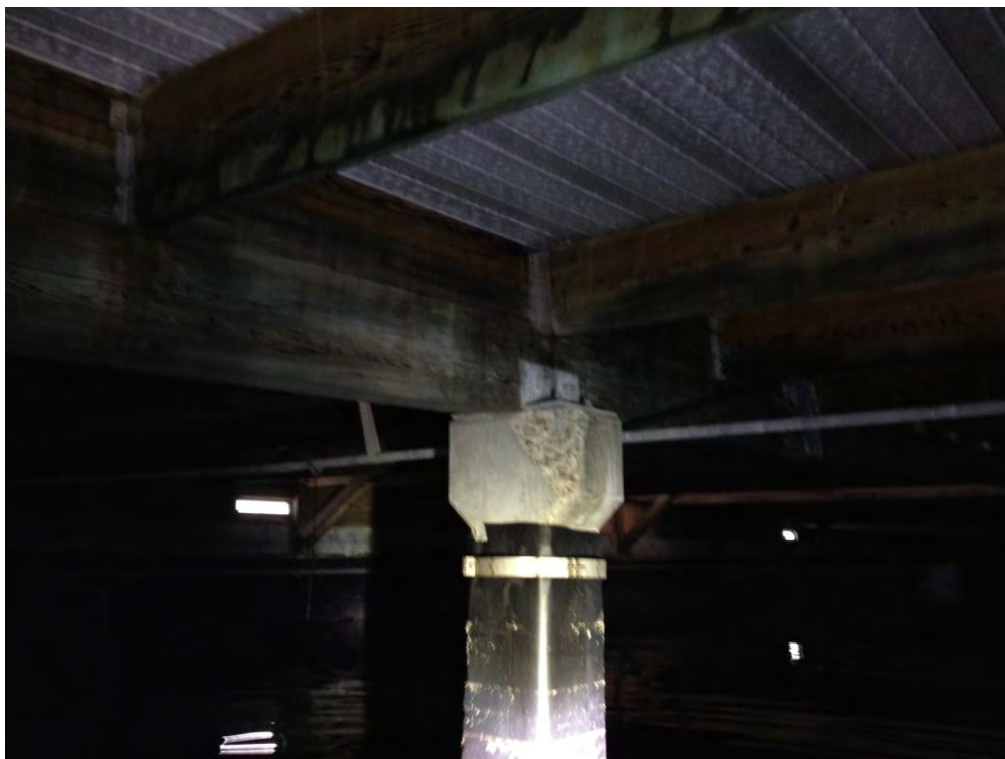
CONCRETE COLUMN WITH BROKEN CORNER
