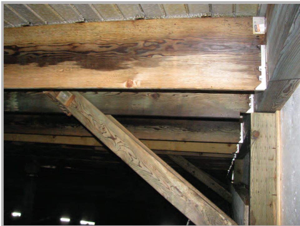
Photo B.8 Peters Canyon Reservoir Typical Purlin and brace at Perimeter Wall
