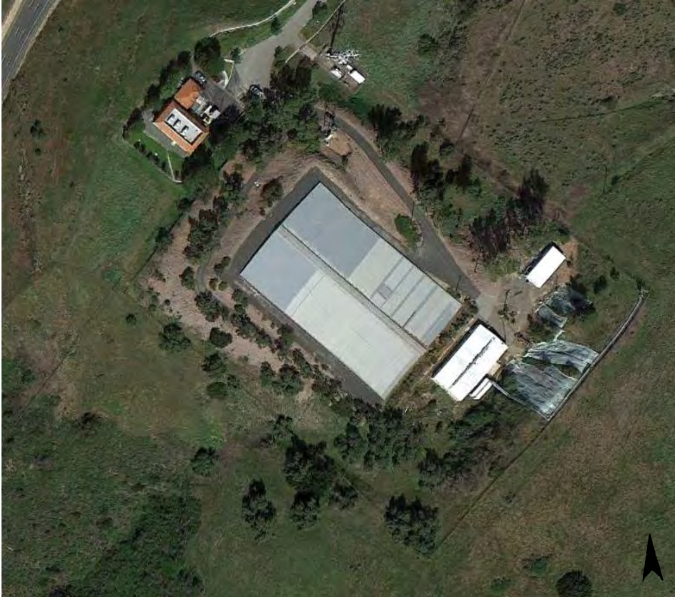
EOCWD PETERS CANYON RESERVOIR
