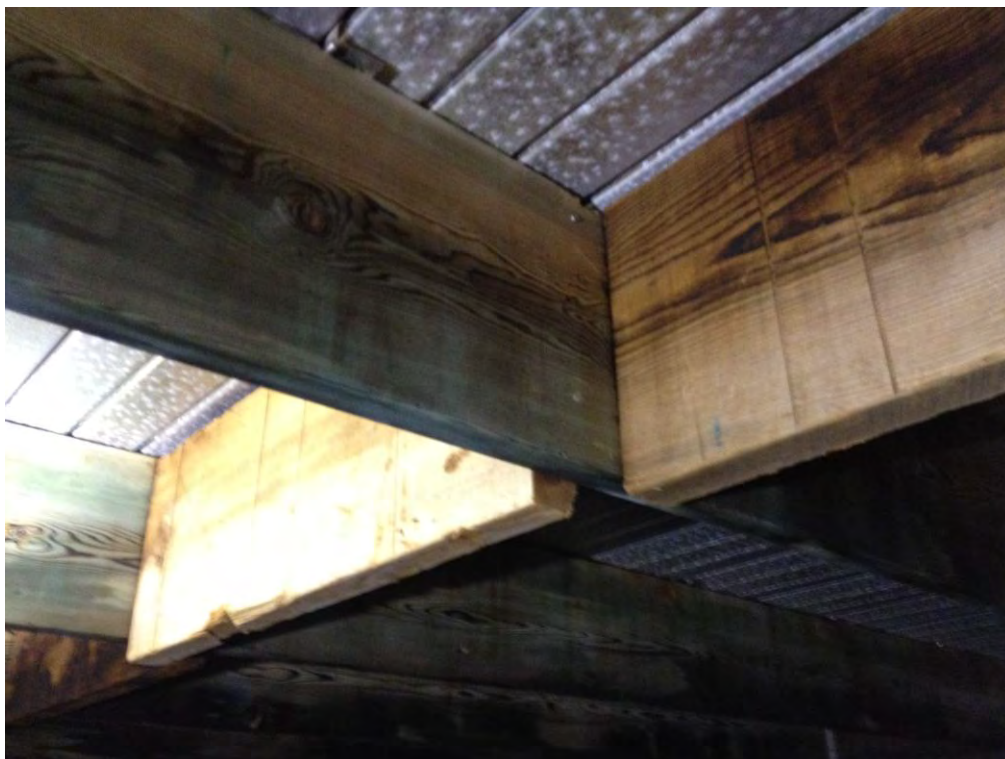
UNDERSIDE OF ROOFING
