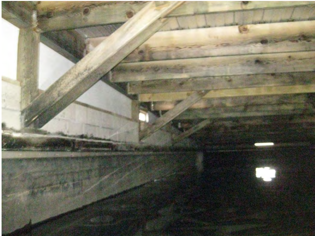
TYPICAL E/W WALL FRAMING
