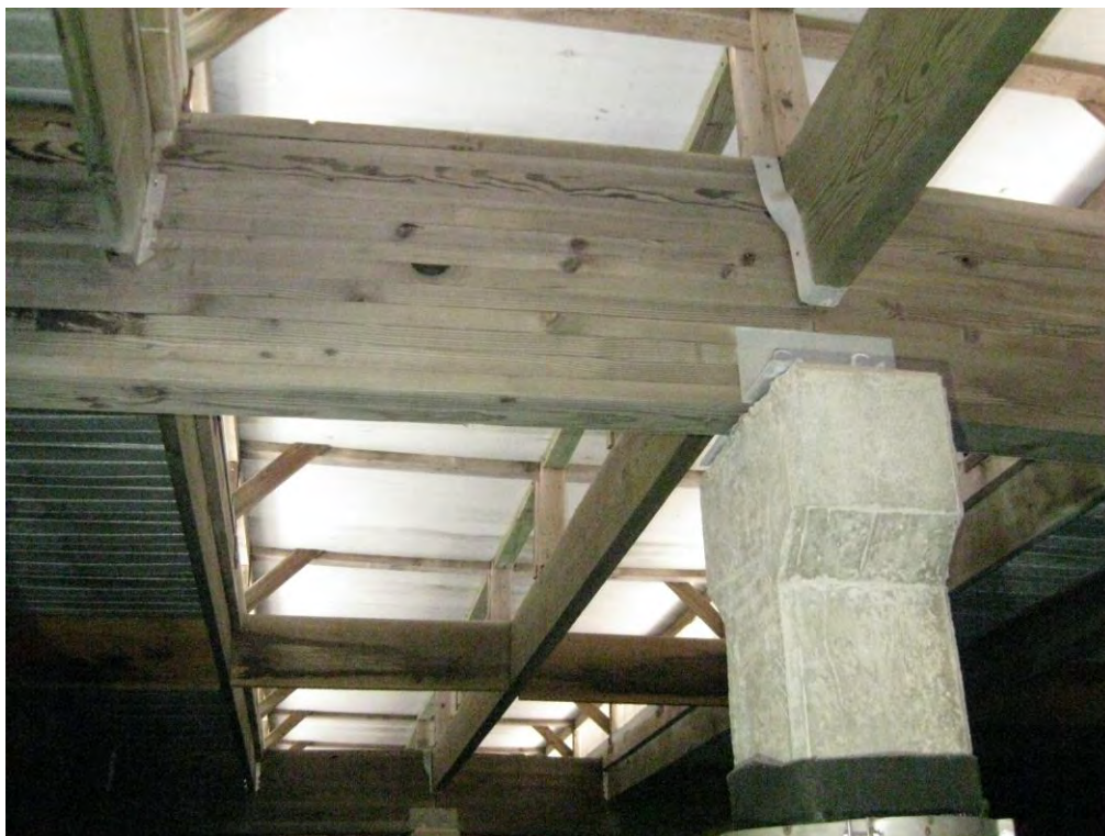
ROOF VENT FRAMING
