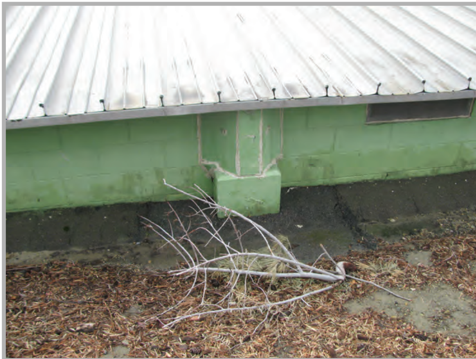
Photo B.4 Peters Canyon Reservoir Typical Pilaster
