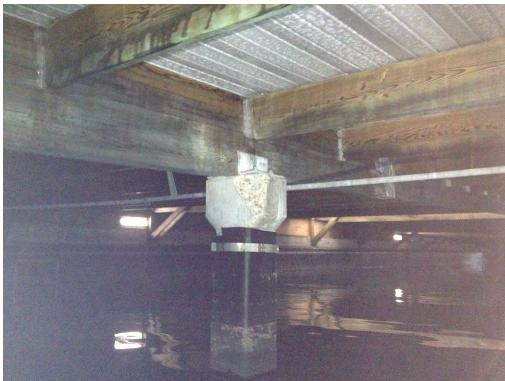
TYPICAL PRECAST CONCRETE COLUMN
