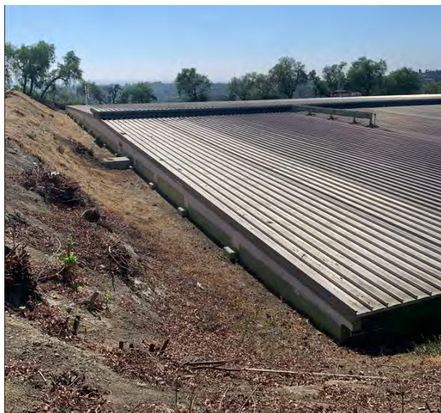
Figure 17 Reservoir Exterior – South End
