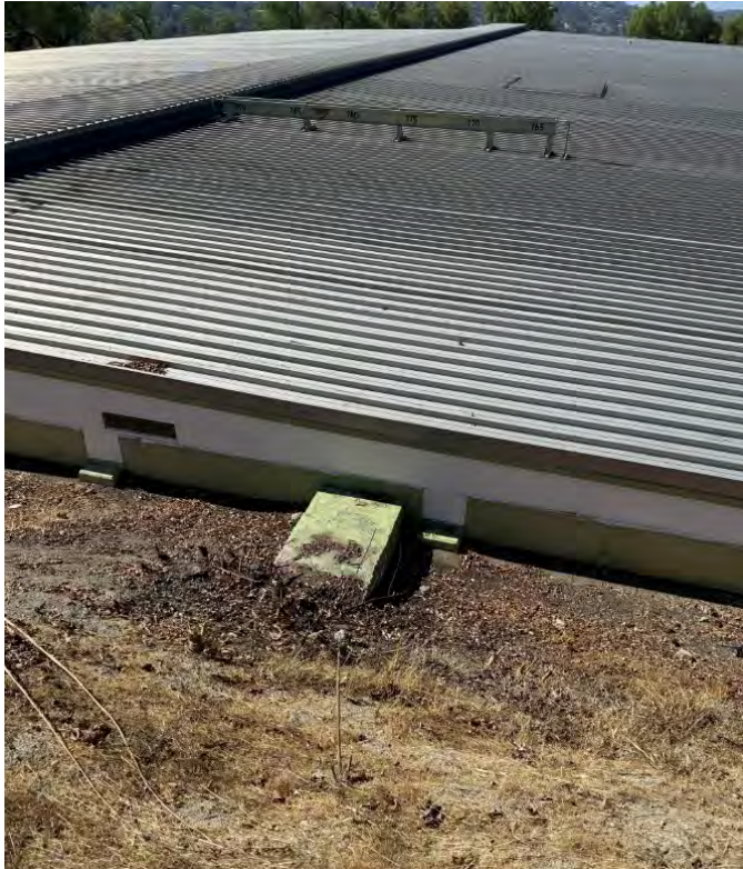
Figure 16 Reservoir Roof and Inlet Pipe – South End
