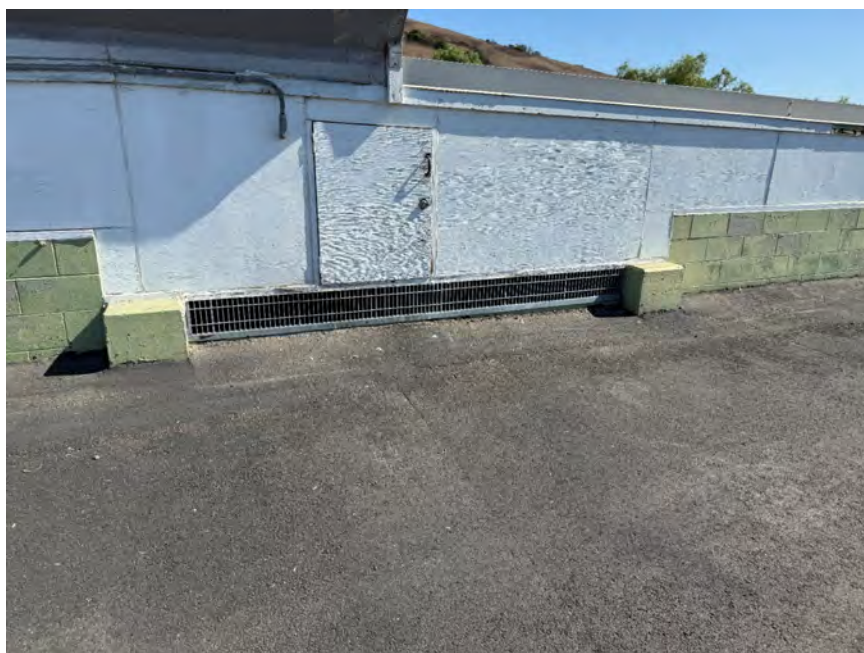
Figure 20 Reservoir Overflow – North End
