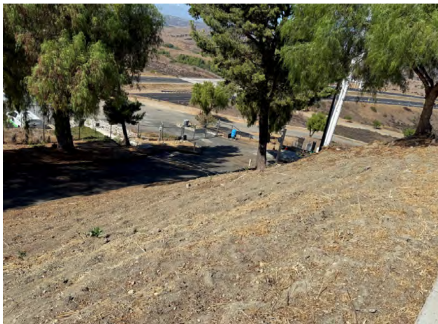
Figure 19 Reservoir Access Road – Entrance Gate
