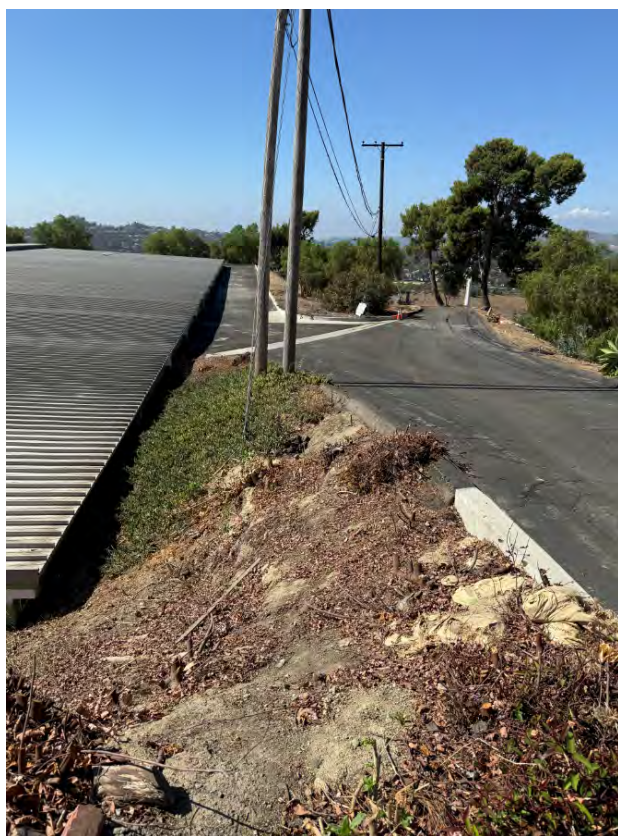
Figure 18 Reservoir Access Road – Looking Northwest
