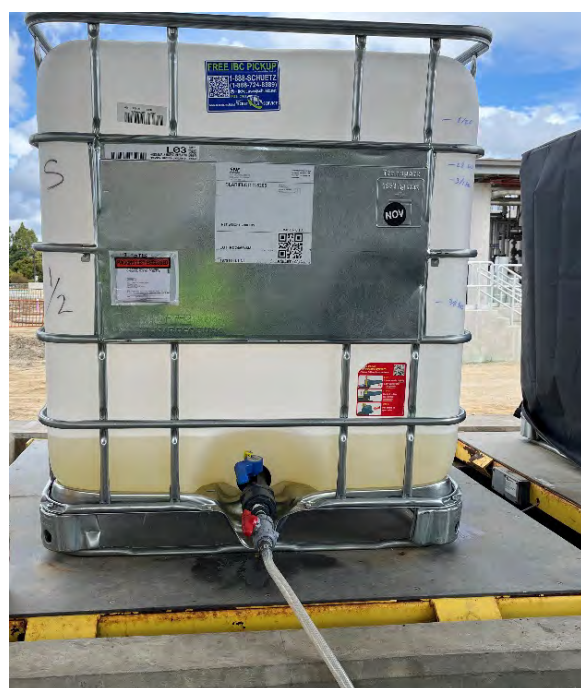
Figure 51 Example of a Chemical Tote Positioned on a Load Cell
