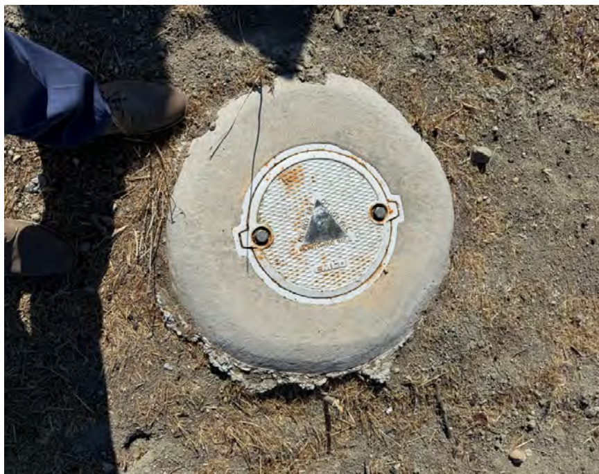
Figure 21 Reservoir Perimeter Monitoring Well
